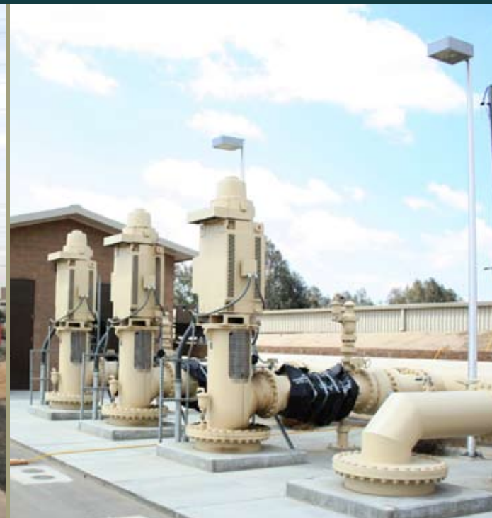
Northwest Pump Station
