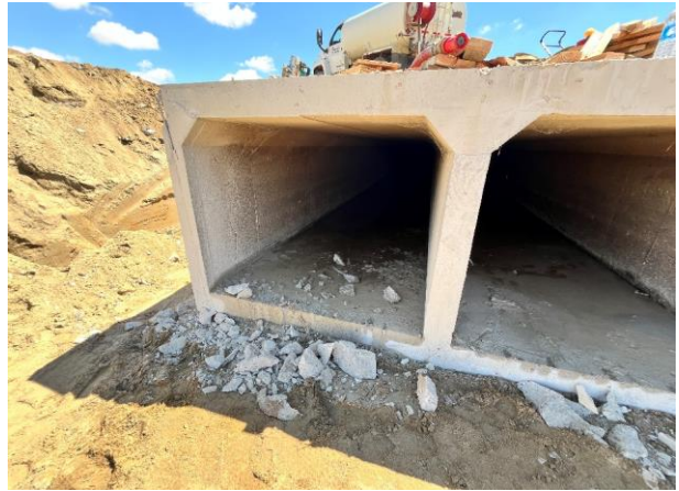
Box culvert sawcut and partially demolished.
