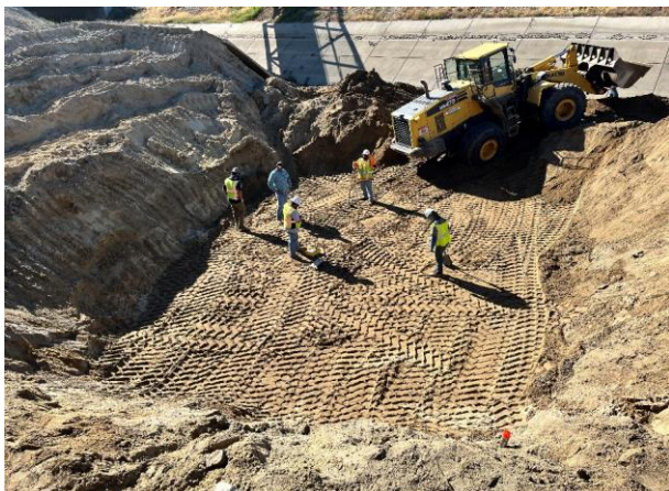
Structure demoed and subgrade work completed.
