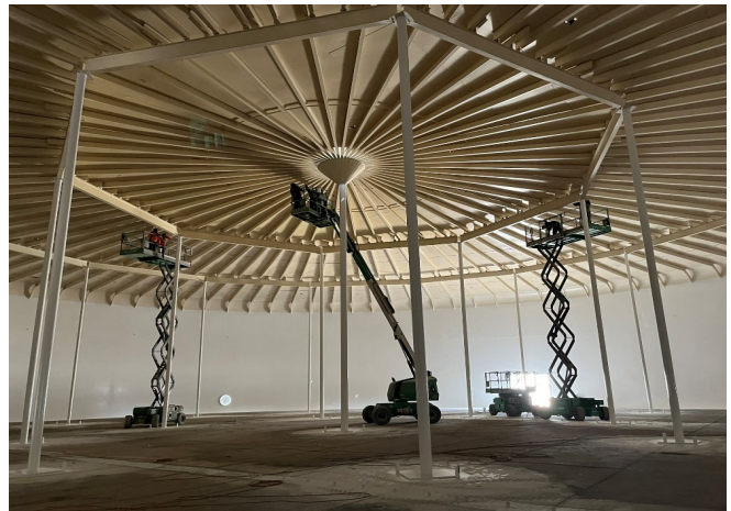
Spot Repairing Interior Roof
