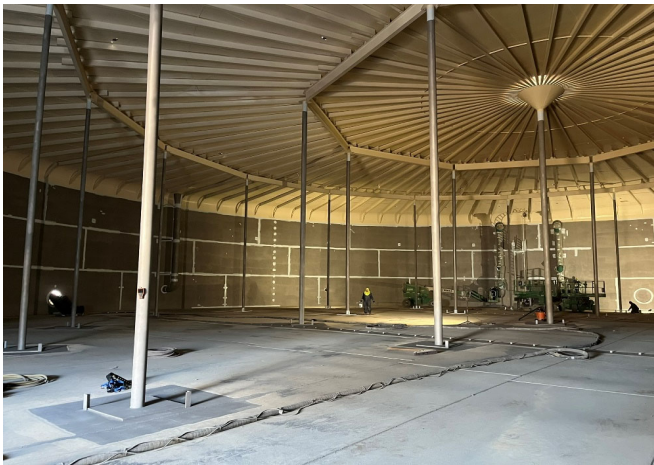
Stripe Coating Blasted Interior Shell
