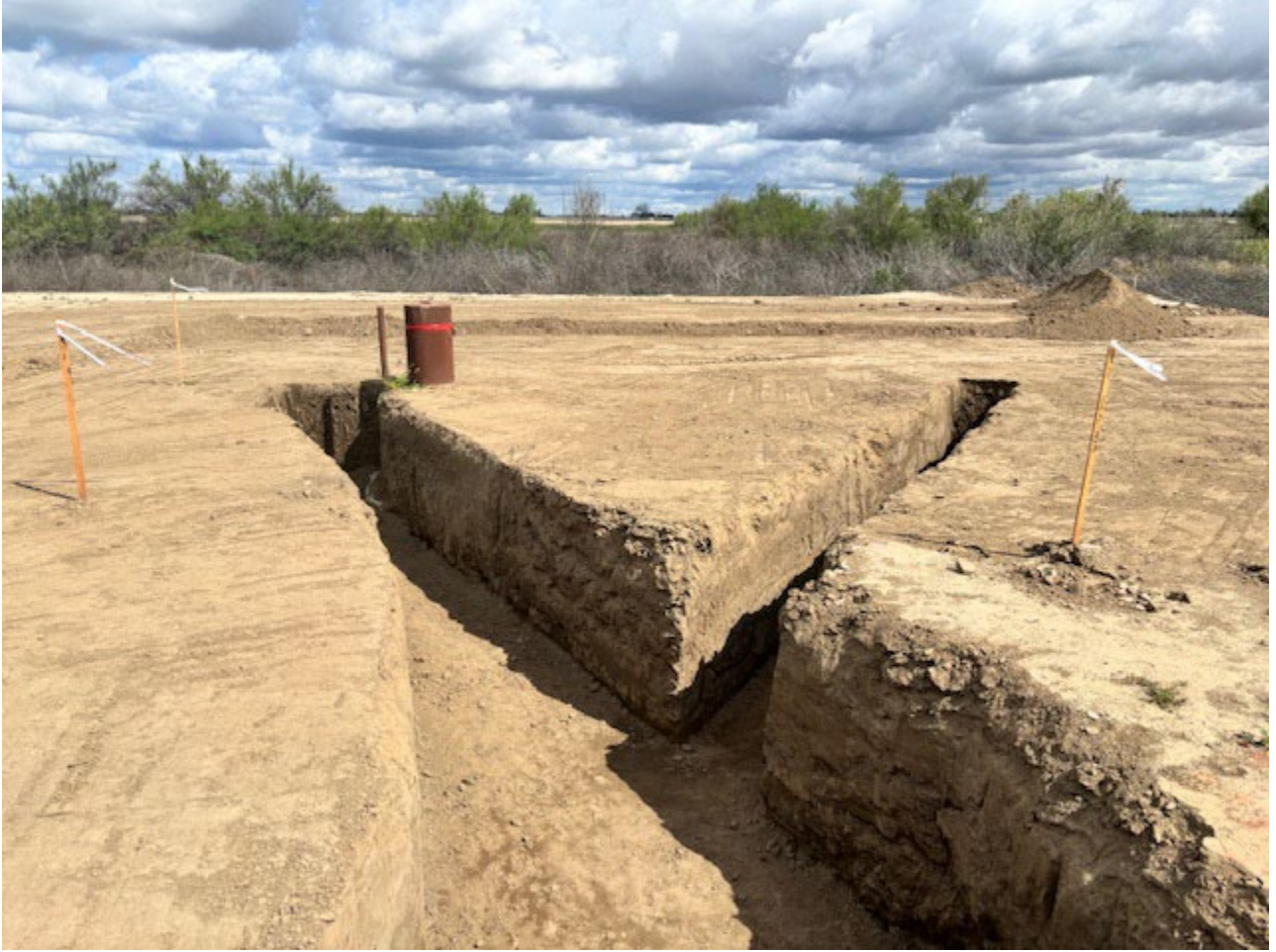
Electrical Conduit Trenches to Well and Well Discharge Piping
