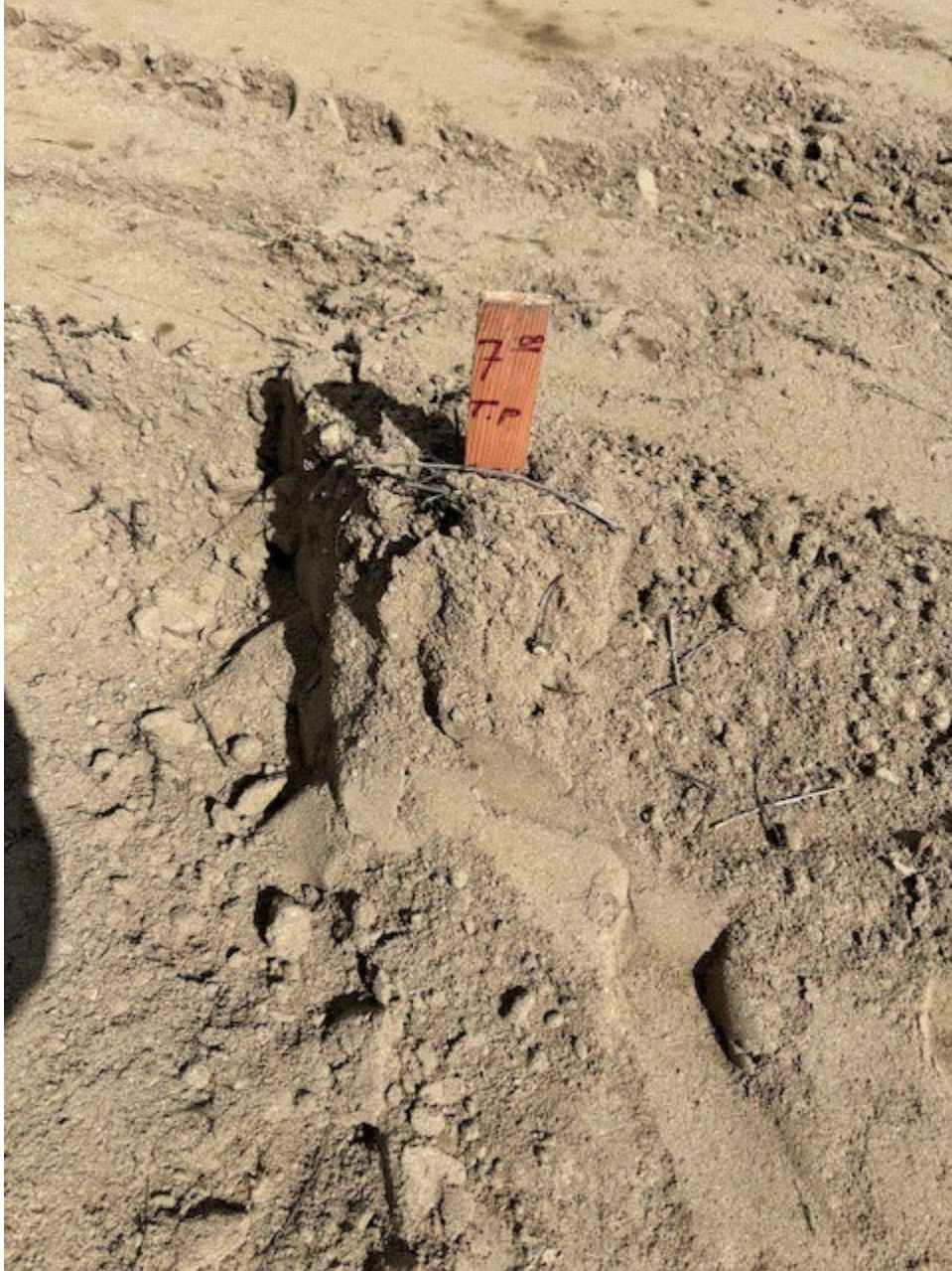
Pothole Location for Existing Pipeline
