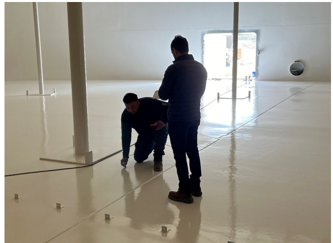
Thickness Testing Interior Coating
