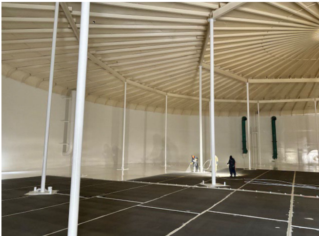
Coating Interior Floor
